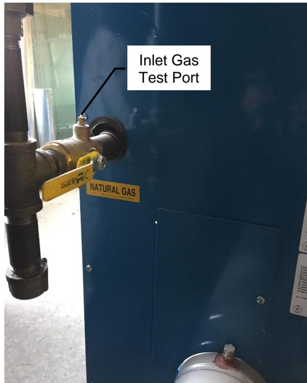
The air flow is pre-set at the factory prior to shipment. Gas flow is dependent primarily on fan speed not upstream gas pressure. The air/gas ratio may have to be adjusted to obtain proper combustion readings for specific local conditions. A combustion analyzer must be used. The probe must be placed in the exhaust vent immediately after the appliance. Combustion should be adjusted in accordance with Table of Combustion Exhaust Settings.
