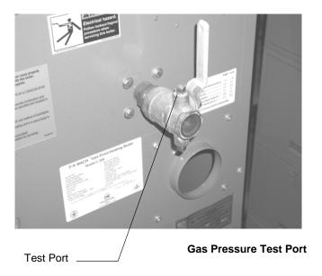
The supply pressure during main burner operation must be greater than the minimum indicated on the rating plate (3.5". W.C. for natural gas, 7" W.C. for propane).
