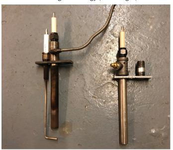
The original flame rod (above left) was producing very inconsistent flame strength signals compared to the upgraded UV scanner which reported a solid 5.0V flame signal at ignition, low fire, and high fire:
