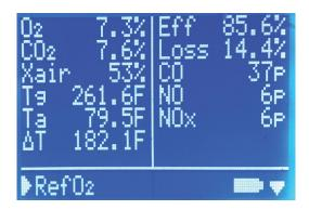
When this water heater left the Patterson-Kelley factory in 1997, its operating efficiency was 85%. 23 years later and this water heater is able to achieve 85.6% efficiency!
