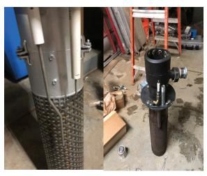
As the flame rod heats up during normal boiler operation, it has a tendency to migrate which reduces the flame signal strength as it moves further away from the burner cylinder. In order to improve the reliability of the flame signal and simultaneously reduce CO and NOx emissions, stainless steel mesh style burners were installed in both boilers, along with an external pilot assembly complete with UV flame monitoring (above right).
